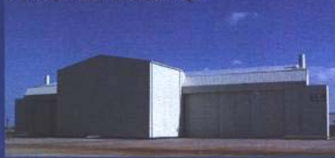
30,000 Square-foot Maintenance Hangar
