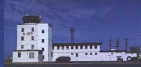
Control Tower with available Office Space
